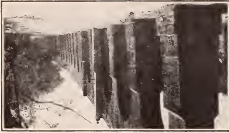
The Aqueduct at Morelia.
